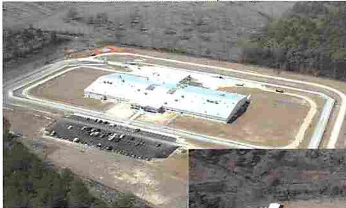
IAH Secure Adult Detention Facility - Phase I
